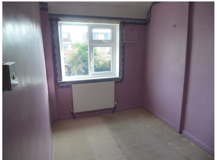
Rear aspect double glazed window, radiator.
